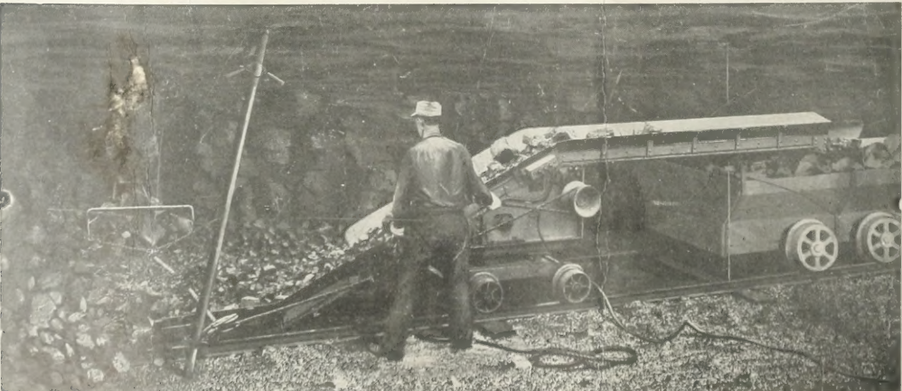
Jeffrey 38-A Pit Car Loader going into low place
